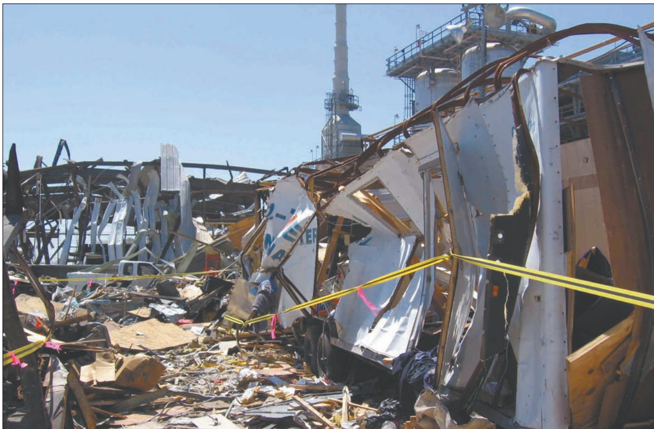
The isomerization unit of the BP America Texas City refinery experienced serious damage after a March 2005 explosion and fire.
