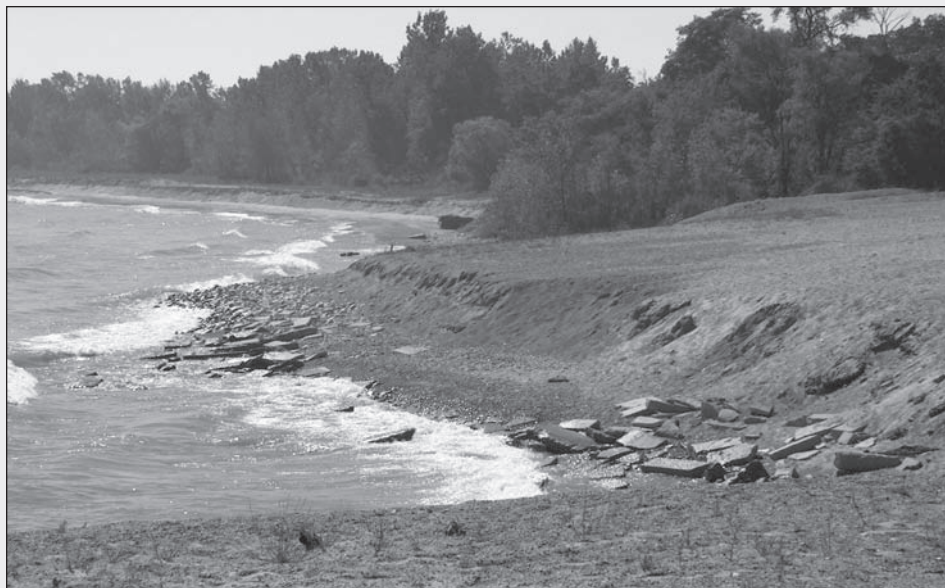
Building materials at North Unit, Illinois Beach State Park.
