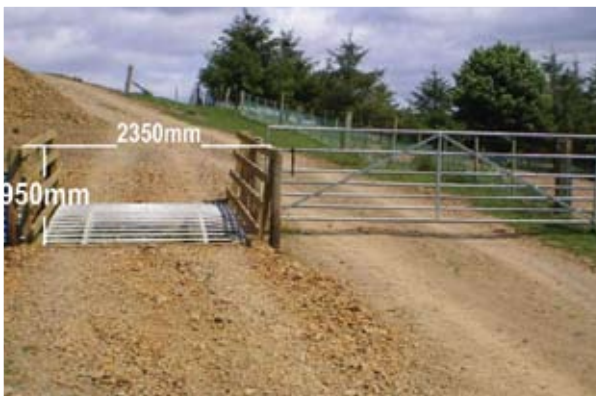
Bike ramps reduce the labour cost of opening and shutting gates
