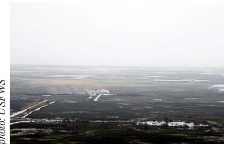
Broken gas well head spews fumes following Hurricane Rita on September 25, 2005 near Sabine NWR.
