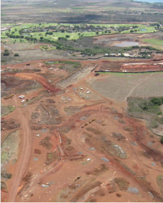
Land clearing for coastal development leads to increased sedimentation on coral reefs delivered in stormwater runoff. Source: NOAA (credit: J. Kozłowski)
