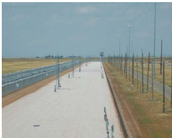
PIDAS (Perimeter Intrusion Detection Access System).
