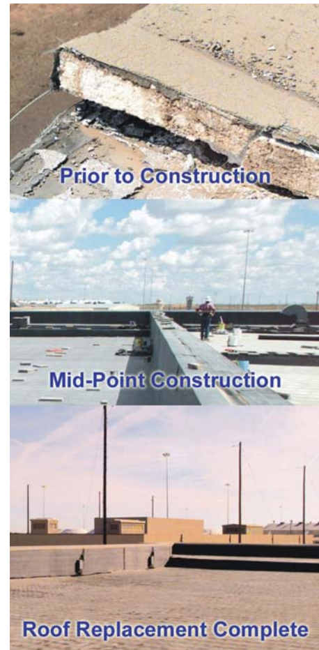
Example of FIRP roof replacement at the Pantex Plant.
