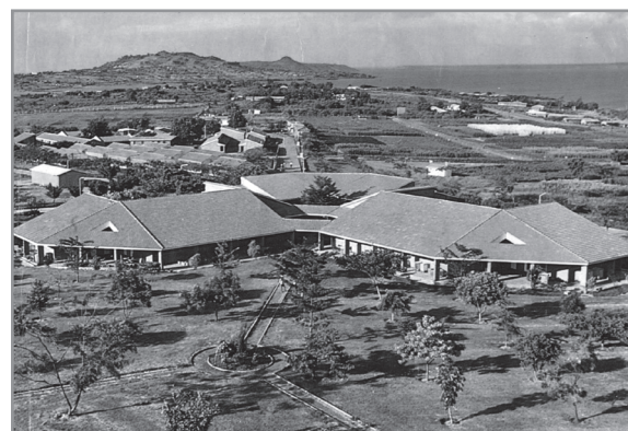
Figure 3. Mbita Point Research and Training Centre on the shores of Lake Victoria, Kenya (ICIPE).
