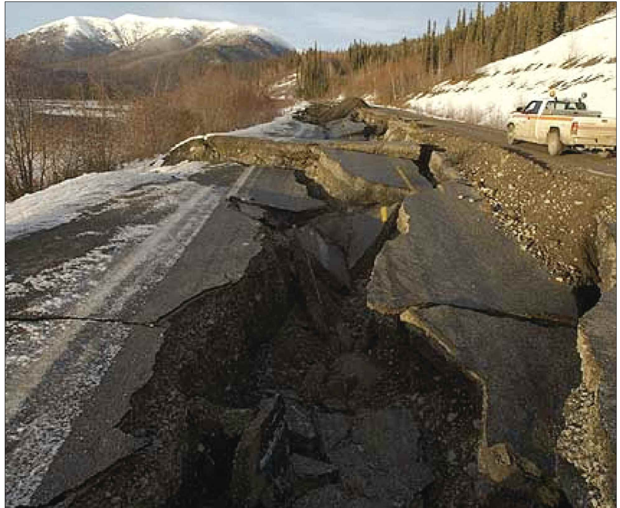
This rupture of the Tok Cutoff Highway in Alaska resulted from a magnitude 7.9 earthquake along the Denali Fault in 2002. The earthquake disrupted roadways and triggered thousands of landslides, but because of the sparsely populated terrain, no one died. (Courtesy Alaska Department of Transportation and Public Facilities)
