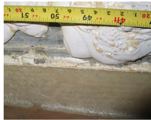
Figure 23: Crack in shear web to LP skin bond joint at 1.20-1.30 m on the CX-100 blade.
