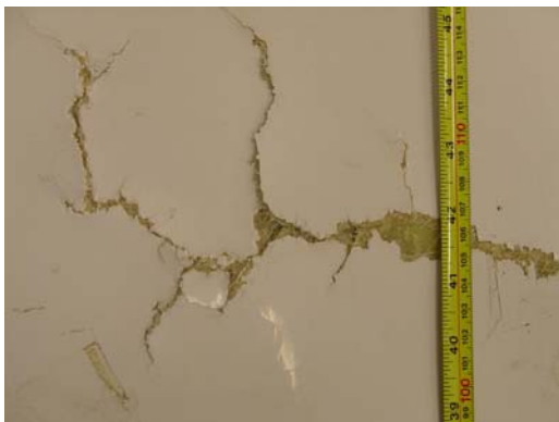
Figure 24: Crack near blade centerline on TX-100 blade.
