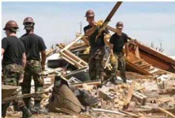
The Kansas Air National Guard works hard to remove debris from Greensburg High School after it was hit by a massive tornado May 4.
