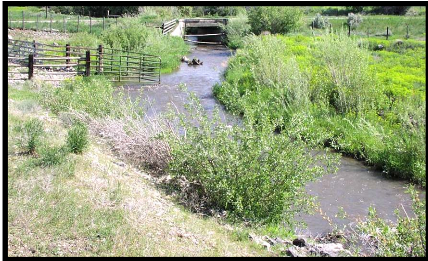
Figure 1: Willow clumps installed in rip-rap along the lower end of Medicine Lodge Creek about 15 miles West of Dubois, ID in August, 2000.
