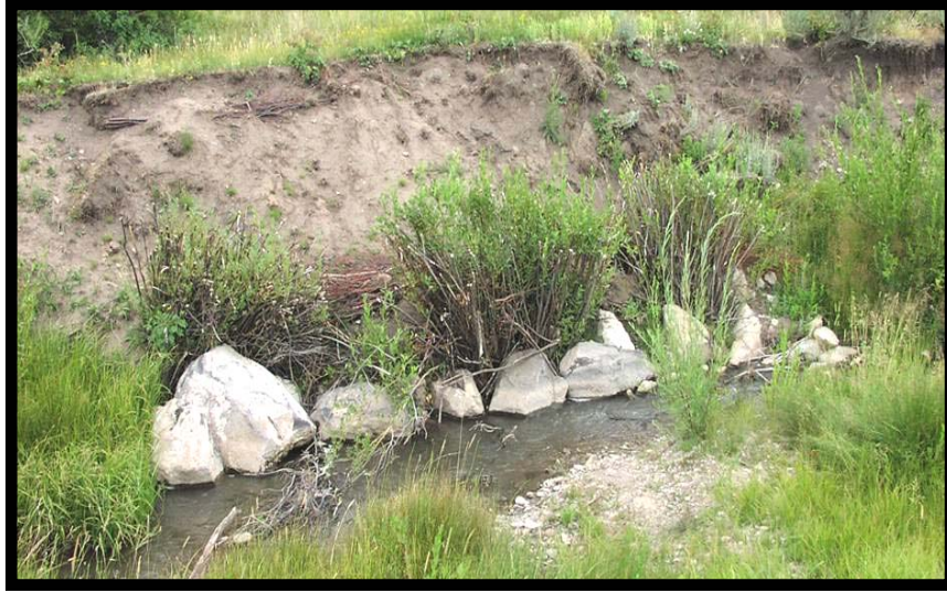
Figure 4: Willow clumps installed on Irving Creek, a tributary of Medicine Lodge Creek, about 25 miles West of Dubois, ID
