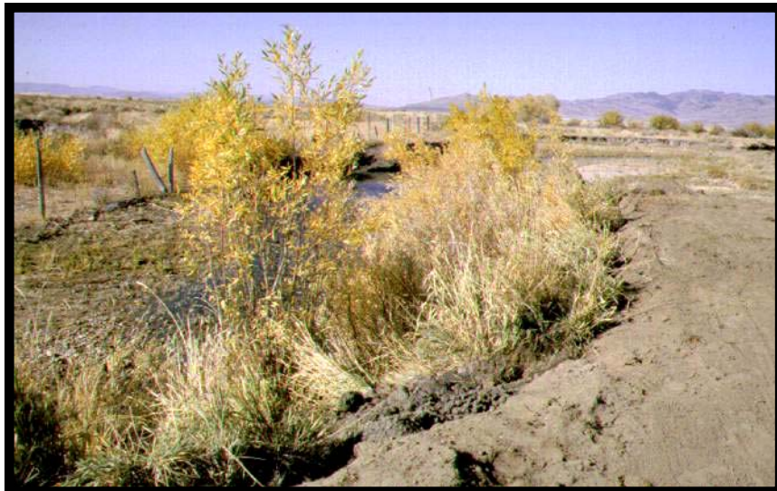
Figure 5: Willow clump planting with sod mats on a streambank of Corral Creek near Fairfield, Camas County, ID
