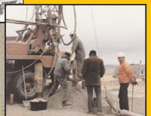
Working with the Laramie Energy Research Center in 1975-1976, Sandia conducted field experiments near Hanna, Wyoming, on in-situ coal gasification. Sandian Dave Northrop is in the orange jacket. Photograph from the Ben Benjamin collection.
