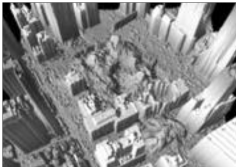
NOAA airborne laser swath mapping (ALSM) image looking southwest over the World Trade Center (WTC). The rubble of 7WTC is at lower right. Behind it are 5WTC (left) and 6WTC (right, damaged). Tower 1 stood behind 6WTC and Tower 2 stood behind and to the left of Tower 1. A wing of 4WTC remains standing at the left-rear of the site.
