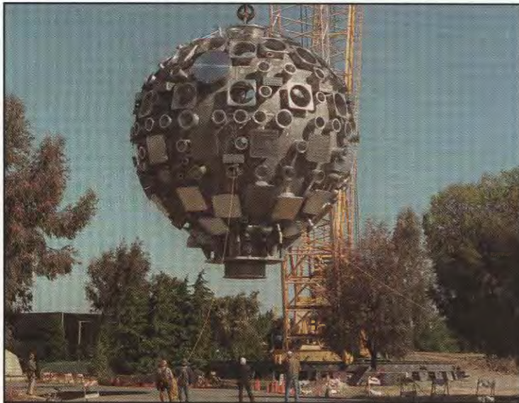
The 192-beam National Ignition Facility during construction in 2001 (top). The 10-meter-diameter target chamber (above and right) was moved into the facility in 1999.
