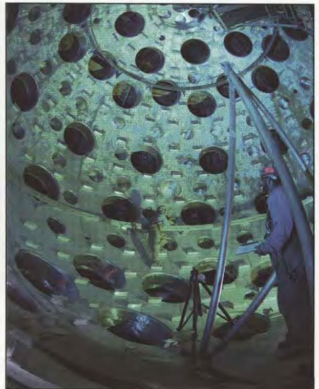
The 192-beam National Ignition Facility during construction in 2001 (top). The 10-meter-diameter target chamber (above and right) was moved into the facility in 1999.
