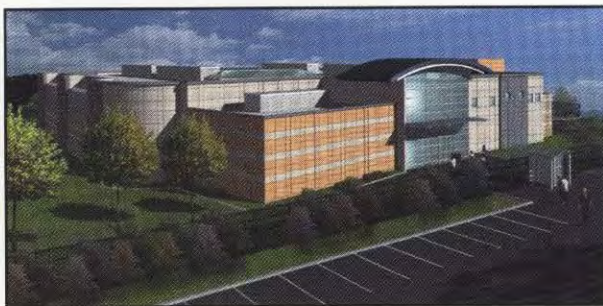
Construction began in 2002 on the $25-million International Security Research Facility, which will consolidate Livermore's nonproliferation and intelligence-related operations into a single building with cutting-edge information technology tools.
