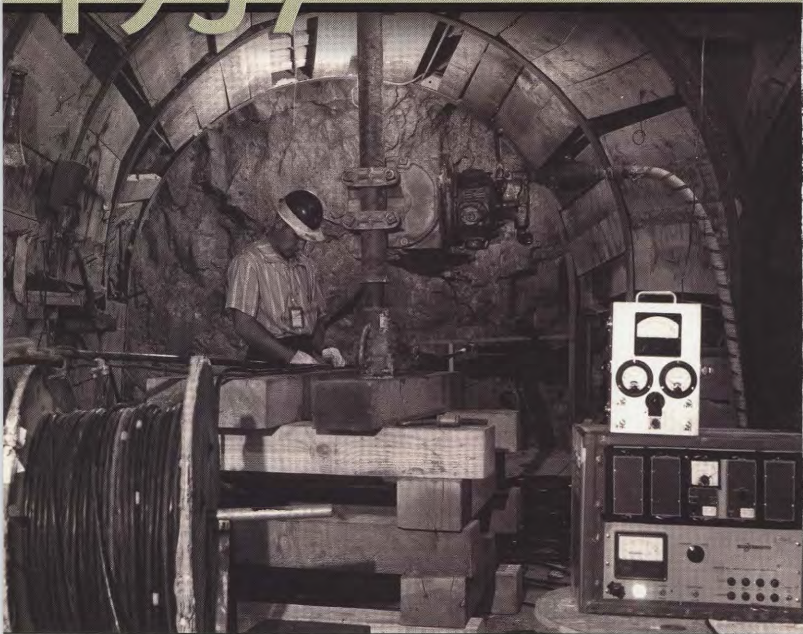
Radiation detection equipment in the foreground monitors the environment for a worker in a tunnel at the Nevada Test Site that was dug for the Rainier event in 1957.
