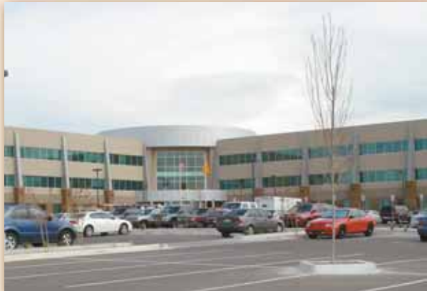
The new IPOC building outside the Kirtland Air Force Base Eubank Gate
