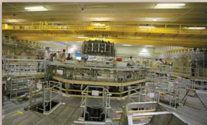
Installation of Z's new center section
