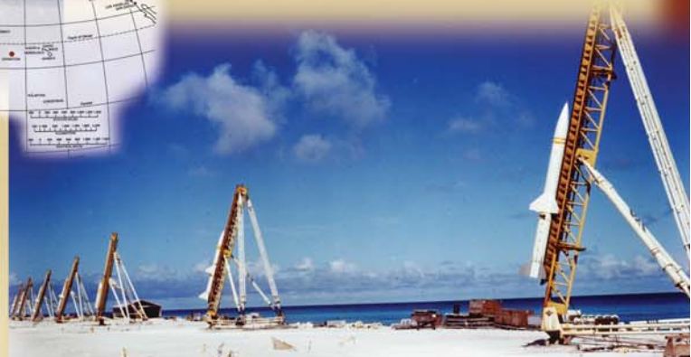
In support of the Teak and Orange events, Sandia designed single- and two-stage Doorknob rockets that were launched from Johnston Island. The rockets measured nuclear radiation, blast, thermal radiation, and electromagnetic effects. Under the leadership of Morgan Kramm, John Eckhart, and Dick Eno, Sandia became a leader in small, unguided rocket design and testing—eventually conducting over 1,500 rocket launches at sites around the world.
