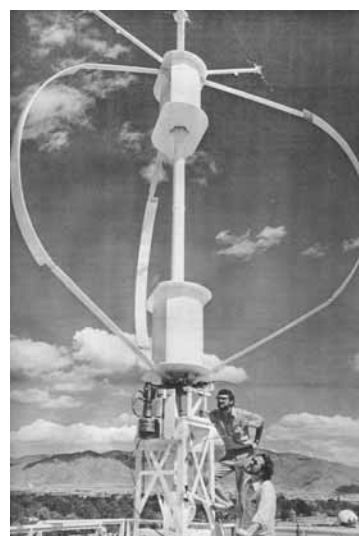
SANDIA'S vertical axis wind turbine, mounted on top of Bldg. 802, in 1974.
