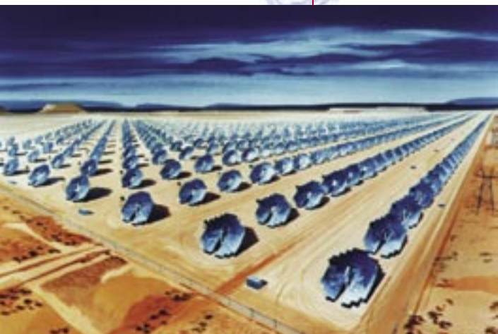
Artist's rendering of a field of dish-Stirling engine systems.
