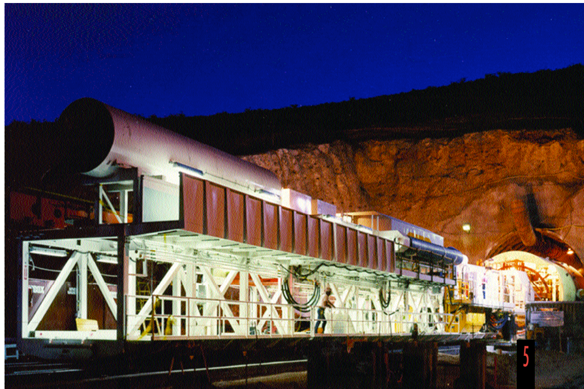
Twilight view of a 25-foot boring machine entering the north portal of Yucca Mountain during drilling of the main drift.
