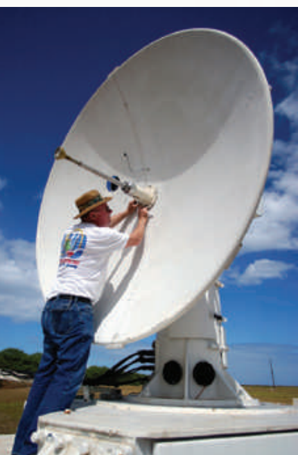
Andy Jones installs a motor assembly on a tracking radar in preparation for a balloon launch.
