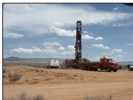
Drilling Operations at SNL/NM
