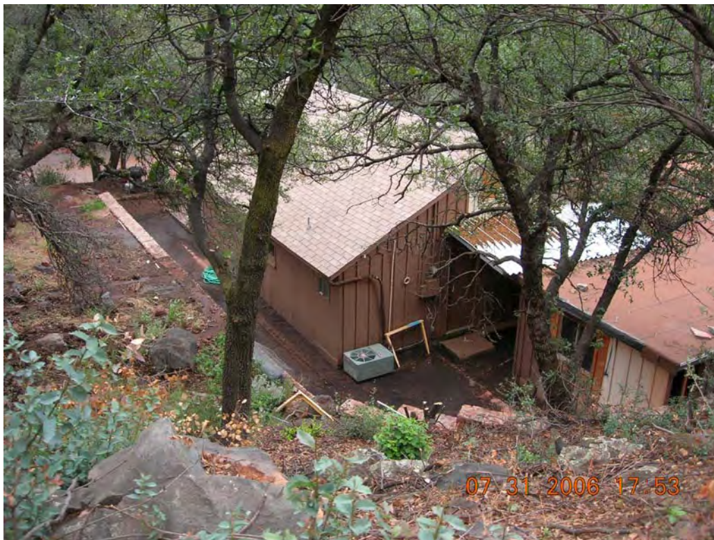
DSCN 1543: Ash and mud deposited in the back of the Dairy Queen. Water and sediment flowed down the slope on the left side of the photo.
