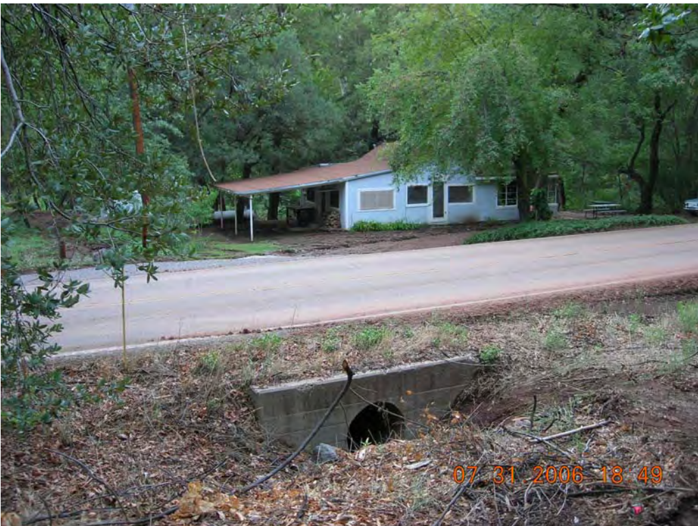
DSCN 1572: Sediment from the debris flow in the above picture was deposited in the front yard of the blue house just south of the Visitor Center area.
