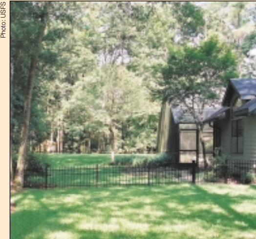
Firewise Demonstration House fencing, before and after the Firewise retrofit. Vegetation has been cleared and the wooden fence attached to the home has been replaced with a metal fence.
