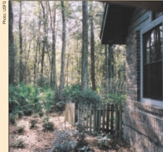
Firewise Demonstration House fencing, before and after the Firewise retrofit. Vegetation has been cleared and the wooden fence attached to the home has been replaced with a metal fence.
