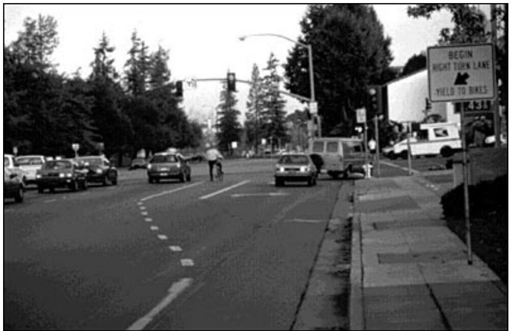
Figure 20. The intersection index increased significantly (indicating a lower level of comfort) if the bicyclist was required to shift to the left to proceed straight through the intersection.
