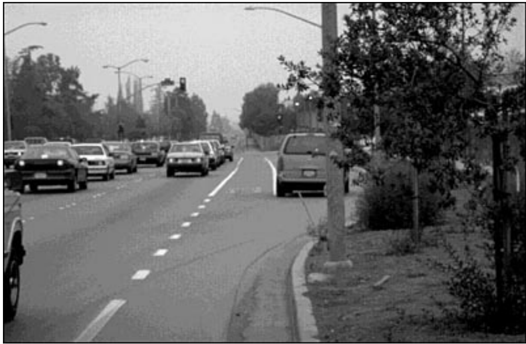
Figure 19. Sites with high volumes of right-turning traffic sometimes contained extremely long auxiliary turn lanes, which made viewing the intersection proper difficult.
