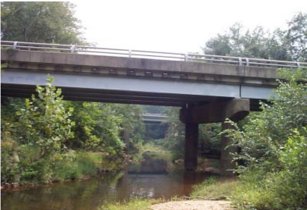
Figure 168. Overall elevation example photograph.
