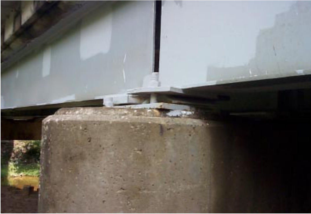
Figure 173. Bearing close-up example photograph.
