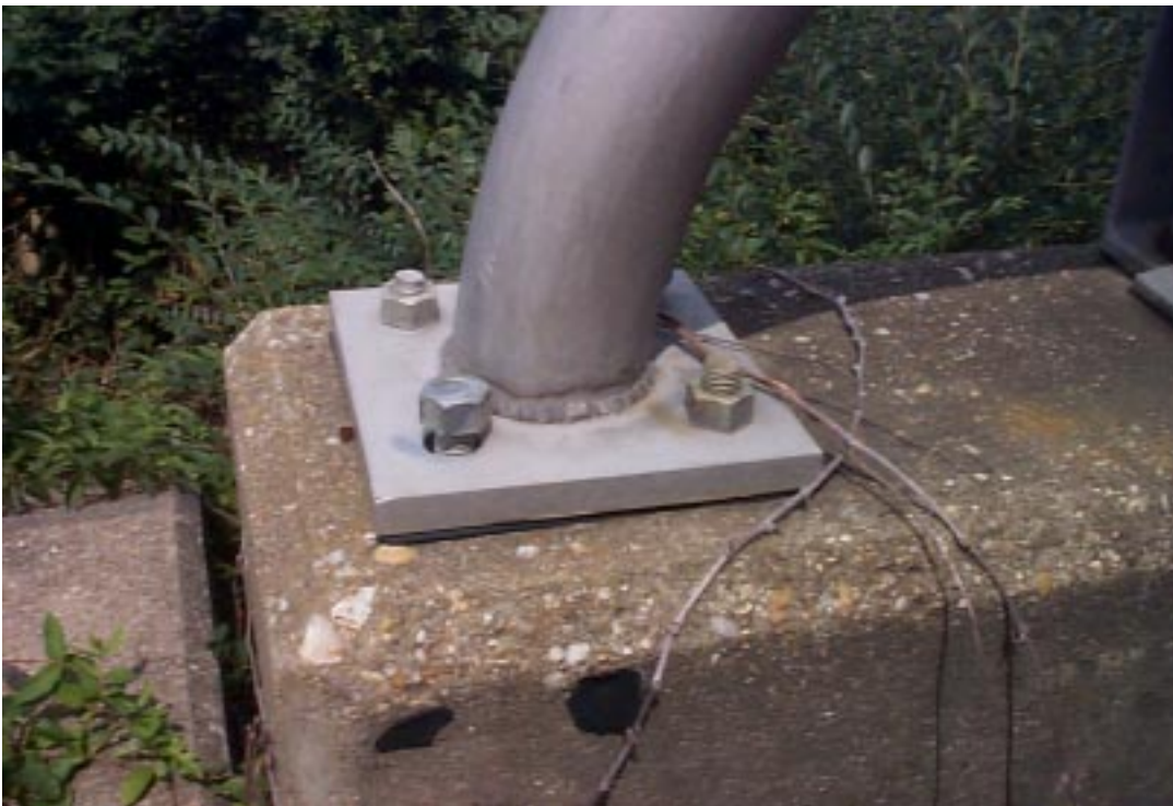
Figure 172. Railing close-up example photograph.
