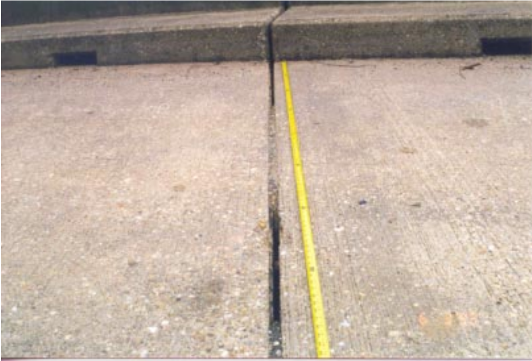
Figure 171. Joint close-up example photograph.
