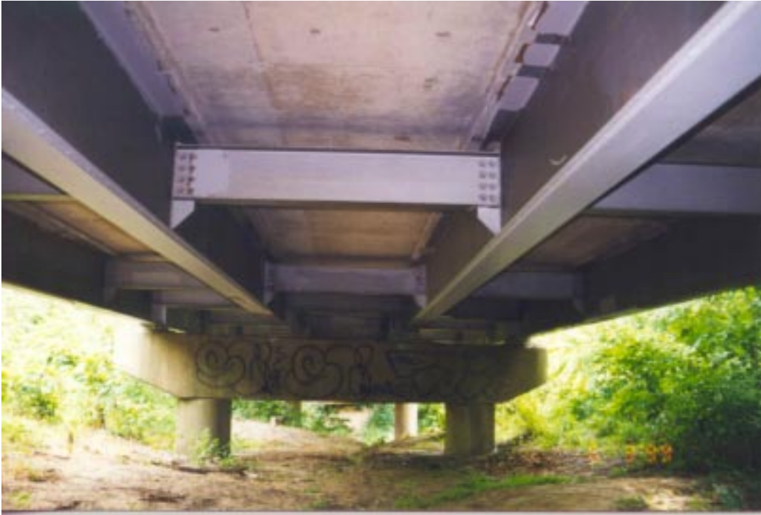
Figure 169. Overall below-deck superstructure and substructure example photograph.
