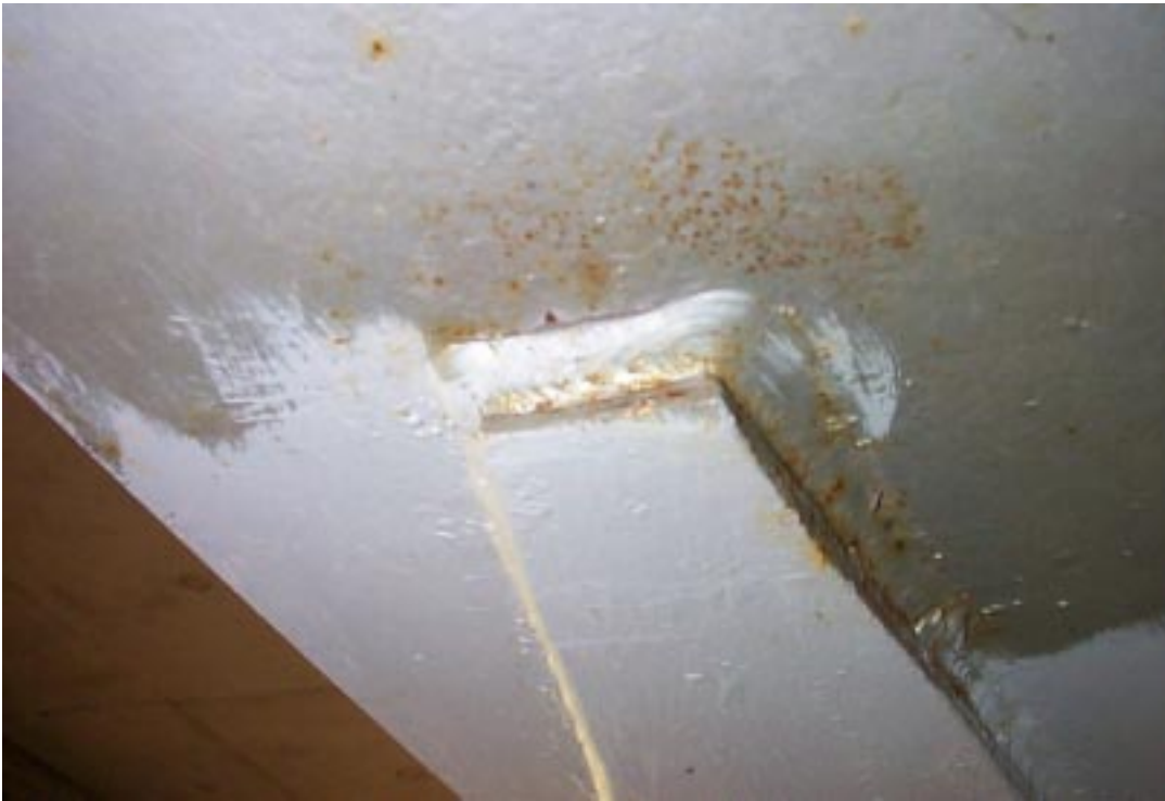
Figure 170. Girder close-up example photograph.
