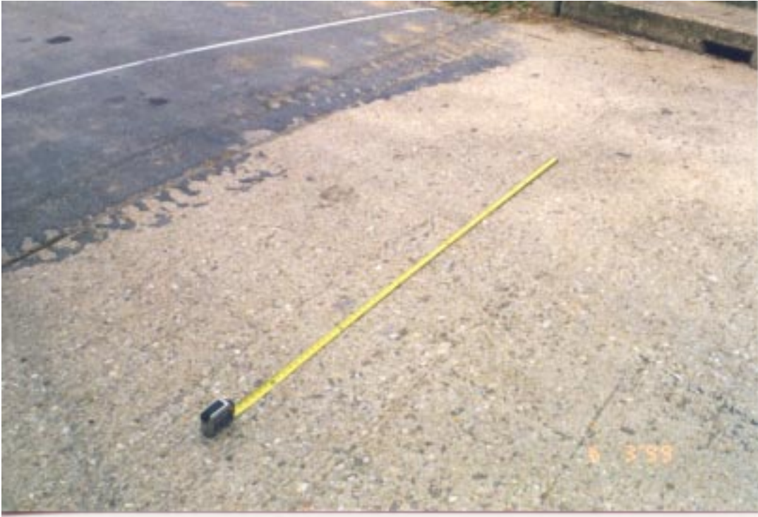
Figure 177. Deck close-up example photograph.
