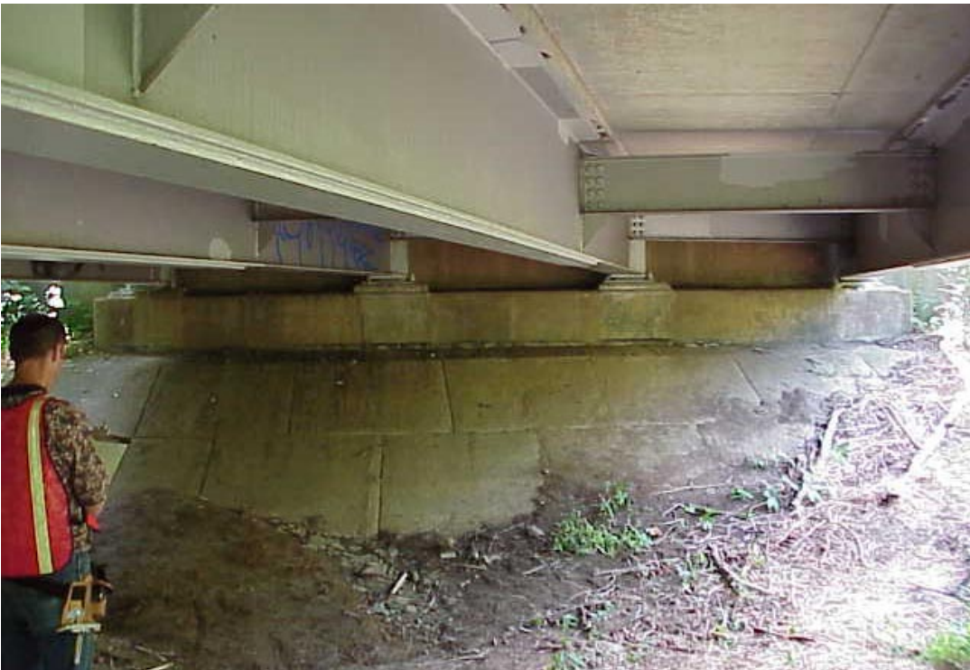
Figure 176. Abutment close-up example photograph.
