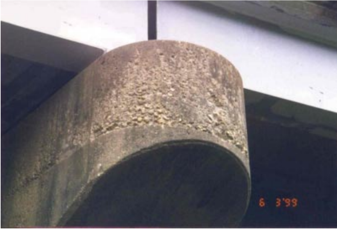
Figure 175. Pier cap close-up example photograph.
