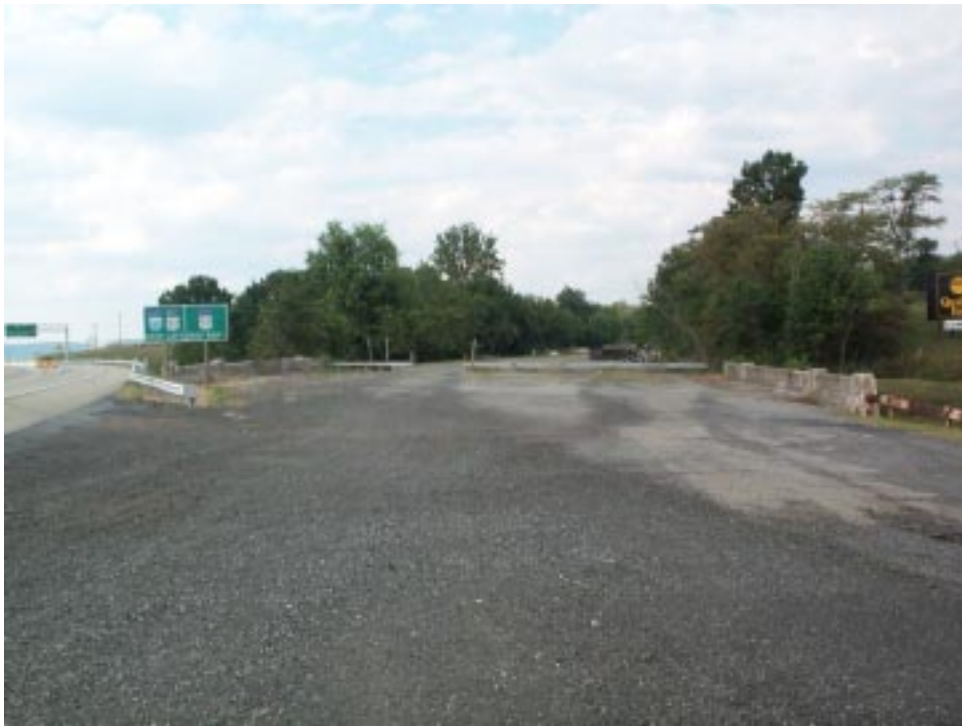
Figure 98. Inspector Photograph 12 – General approach view.
