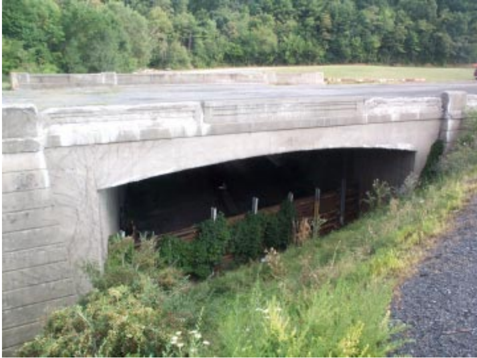
Figure 97. Inspector Photograph 11 – North elevation view.
