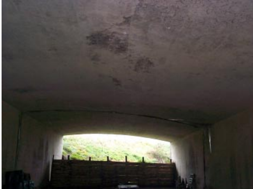
Figure 103. Inspector Photograph 17 – General photograph of bridge underside.
