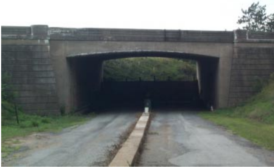
Figure 99. Inspector Photograph 13 – South elevation view.
