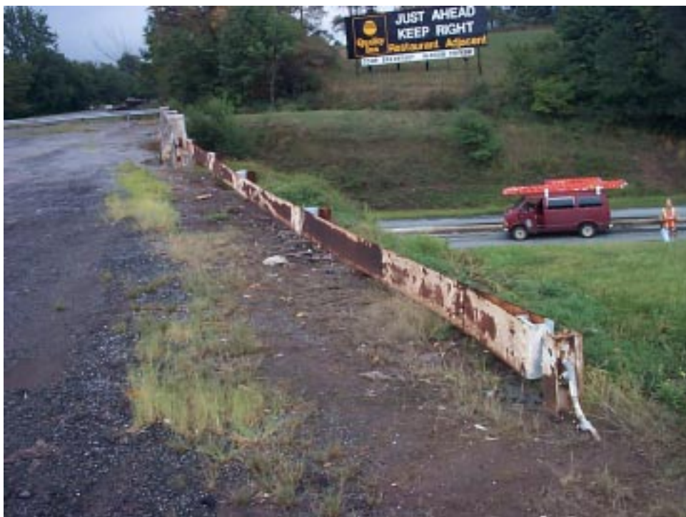
Figure 102. Inspector Photograph 16 – General approach rail condition.
