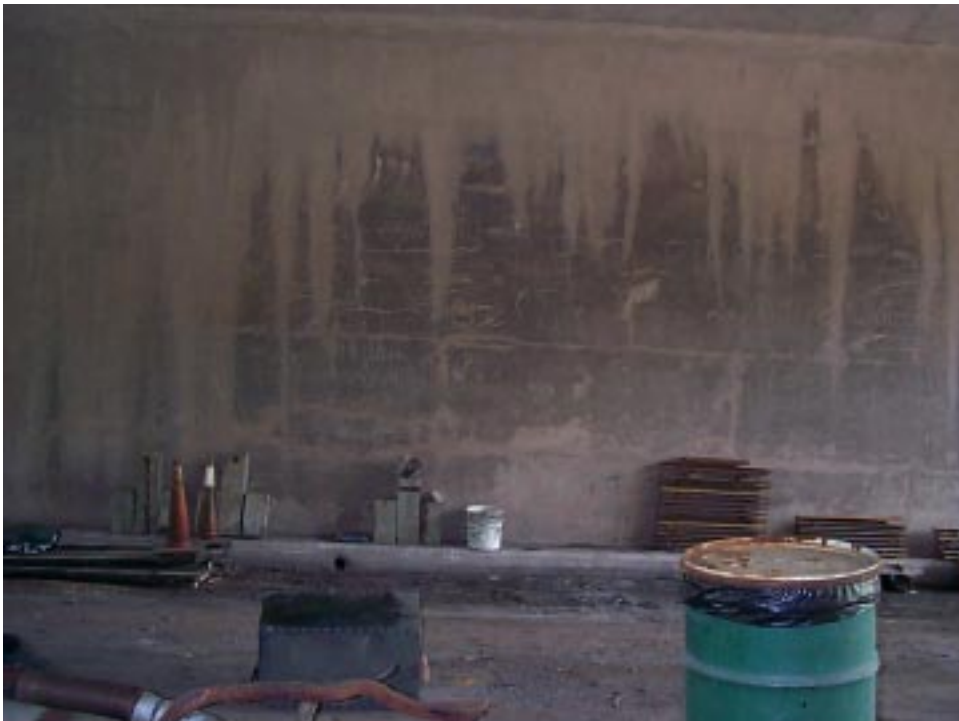
Figure 100. Inspector Photograph 14 – General backwall condition.
