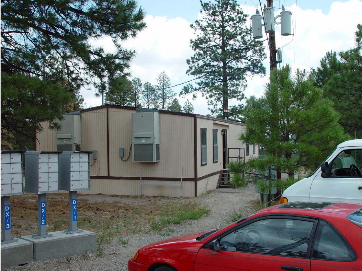
Photo 3. Transportable at TA-69 (Building 2).
