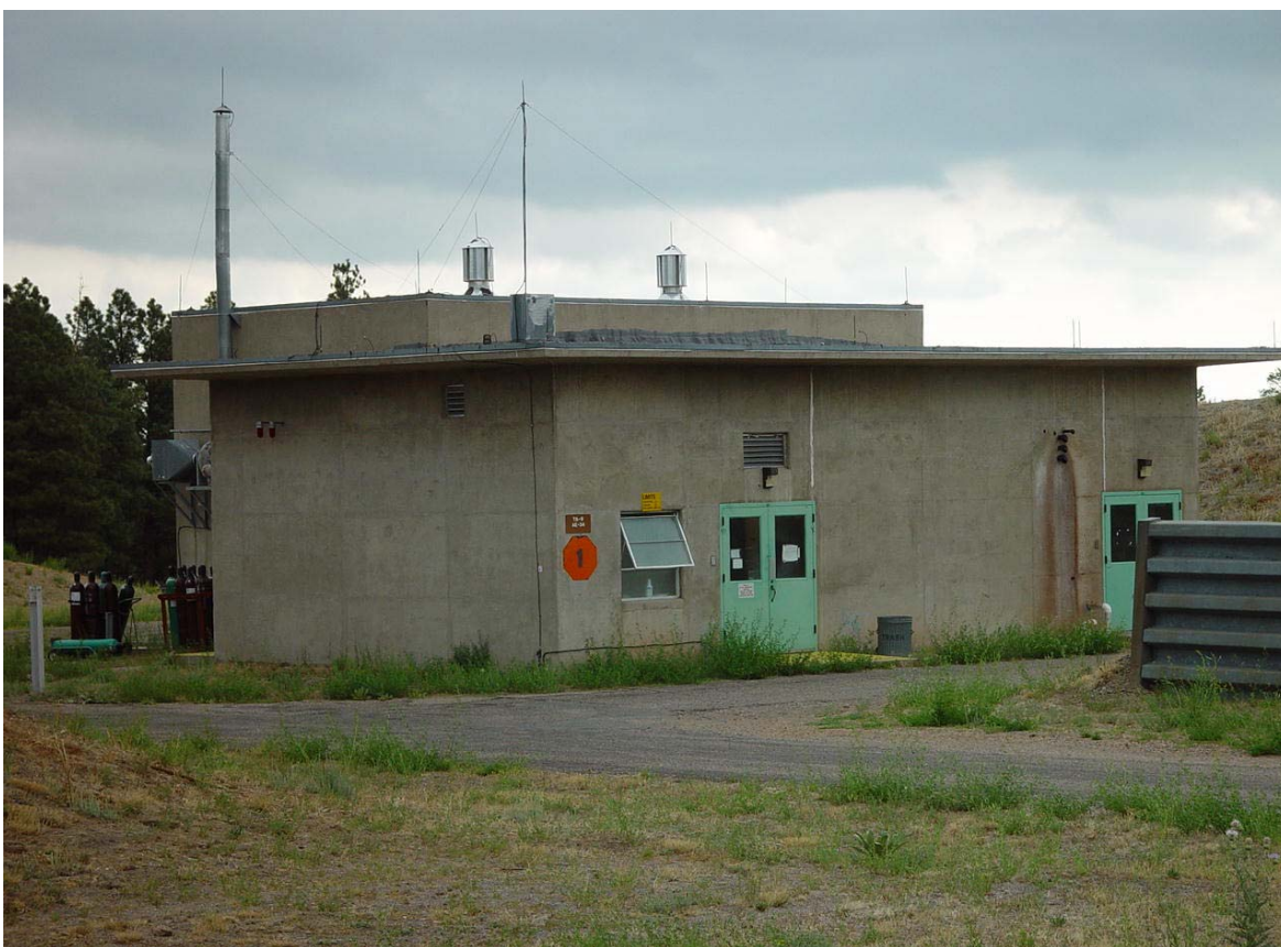
Photo 6. Typical energetic materials research building (TA-9 Building 34).
