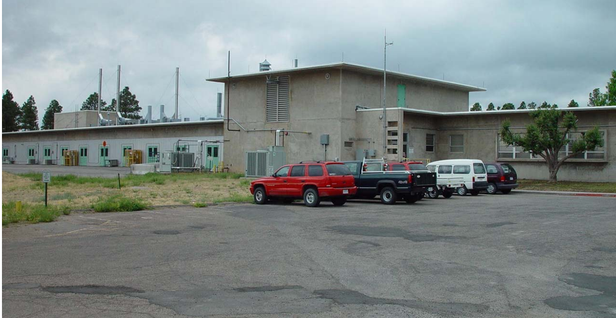
Photo 1. TA-9 Building 21, built in 1952.
