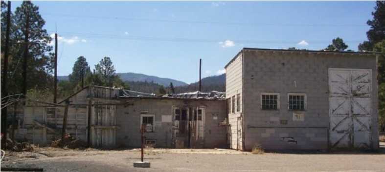
Before and after photos of Building 516 restoration
