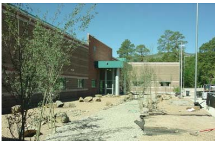
June 08 — Finishing touches are completed
