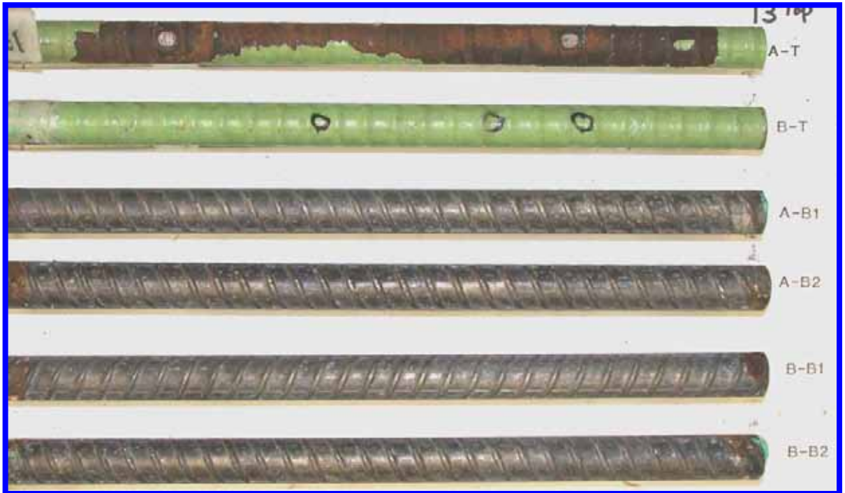
Figure 83. Slab #13 after autopsy
