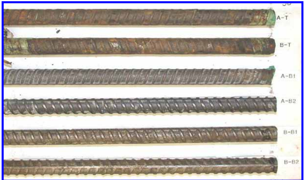
Figure 134. Slab #30 after autopsy
