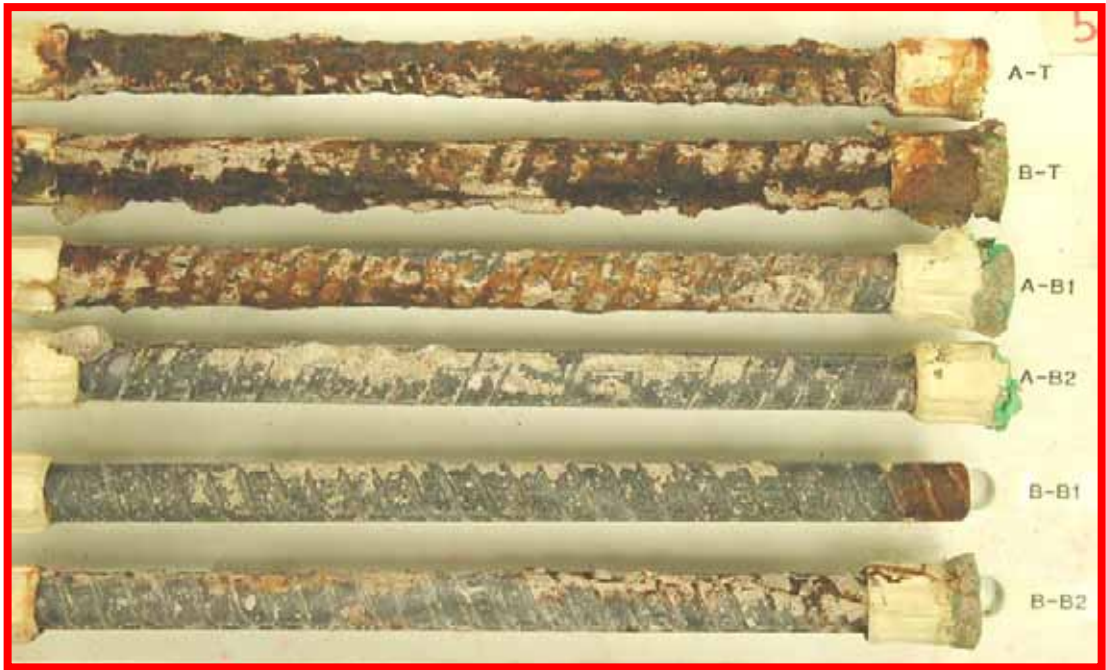
Figure 58. Slab #5 extracted rebar condition
