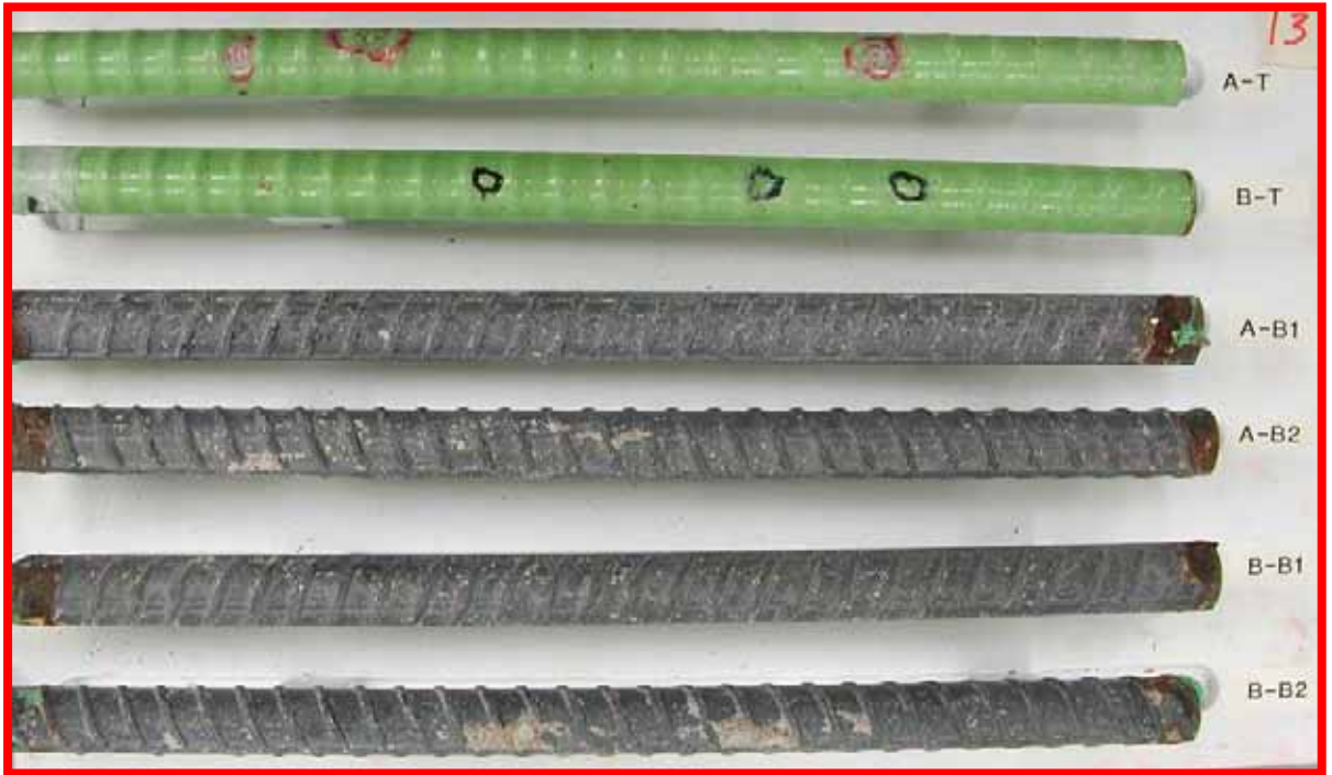
Figure 82. Slab #13 extracted rebars condition
