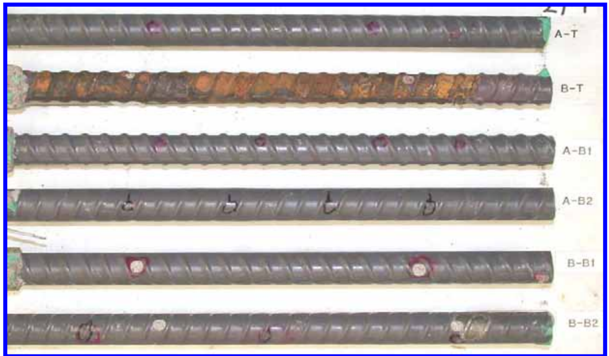
Figure 131. Slab #29 after autopsy
