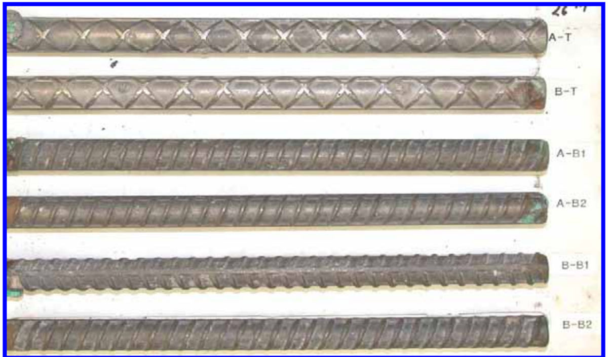
Figure 122. Slab #26 after autopsy
