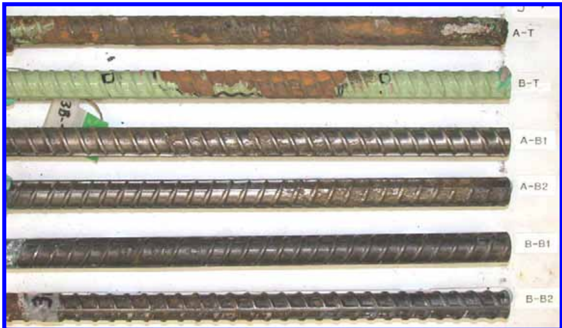
Figure 53. Slab #3 after autopsy
