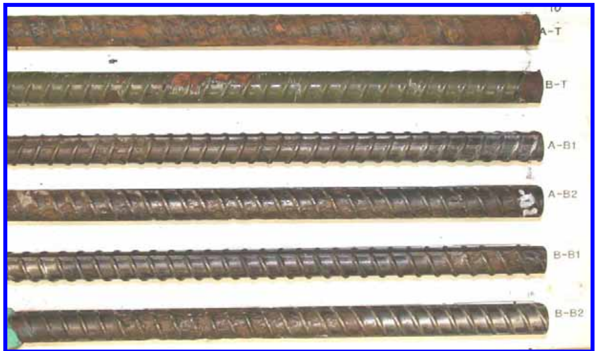
Figure 98. Slab #18 after autopsy
