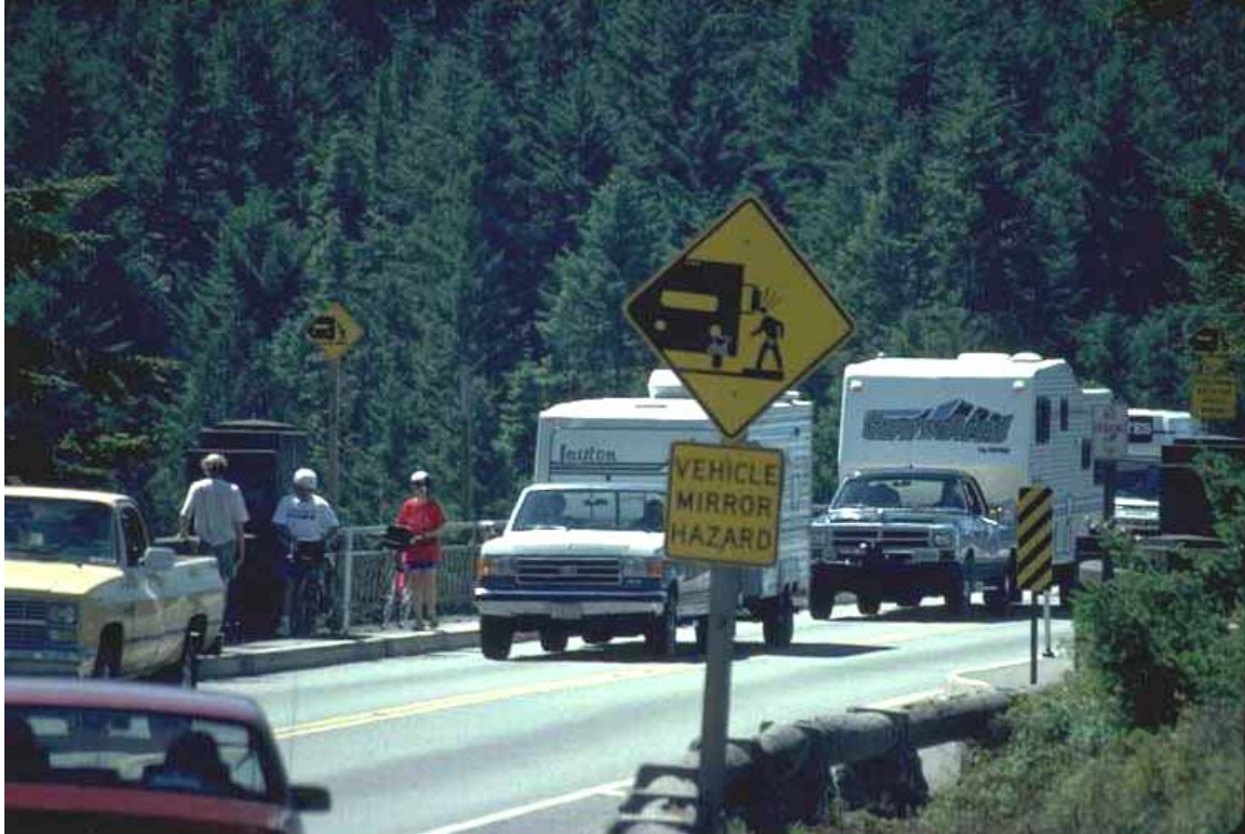
Figure 22-6. Photo. Use of signing to warn motorists and pedestrians of the potential hazard posed by vehicle mirrors on narrow bridge sidewalks.
