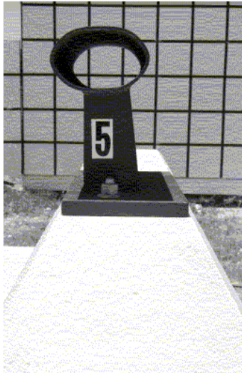
Figure 89. Parapet damage after test P5, side.
