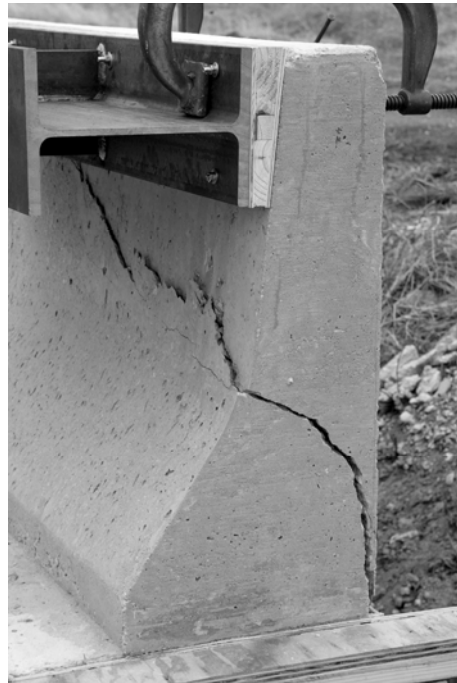
Figure 133. Failure mode at end of the safety-shaped barrier.
