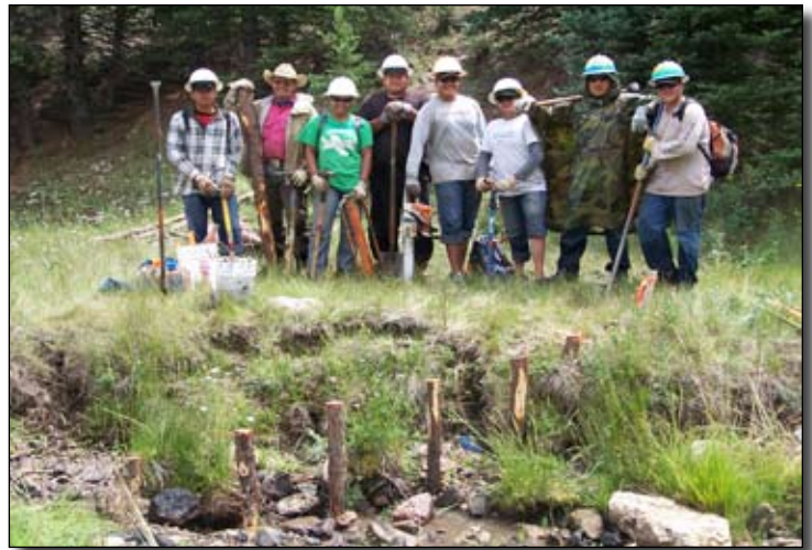
Gallup Youth Conservation Corps helps implement riparian restoration structures along Comanche Creek, July 2006
