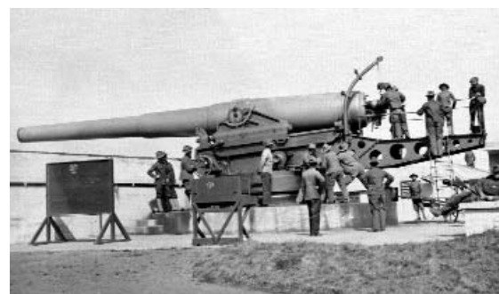
The largest of the new guns installed at the Presidio in the 1890s, like this one at Battery Godfrey, had 12-inch bores.
