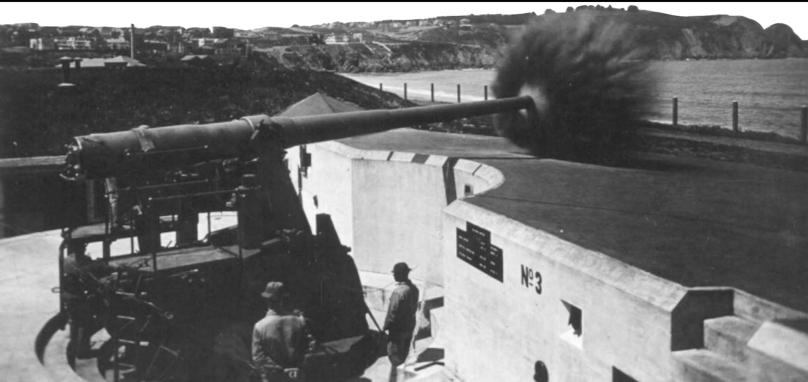
Practice firing of an original 6-inch gun mounted on a disappearing carriage, around 1910.
