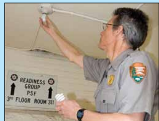
We are replacing incandescent bulbs with compact fluorescent lights in most fixtures.
