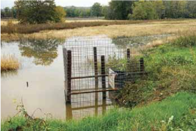
A water-control structure allows the water level to be manipulated when fields are flooded for waterfowl.
