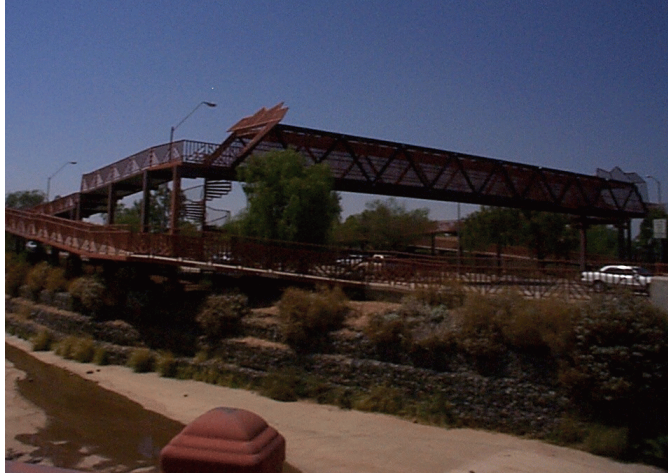
Figure 15. Grade-separated crossings are sometimes used when other measures are not feasible to provide safe pedestrian crossings.
