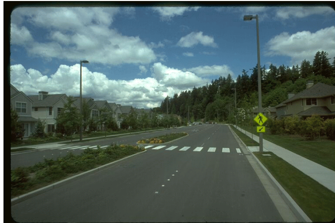
Figure 10. Raised medians and crossing islands can improve pedestrian safety on multi-lane roads.
