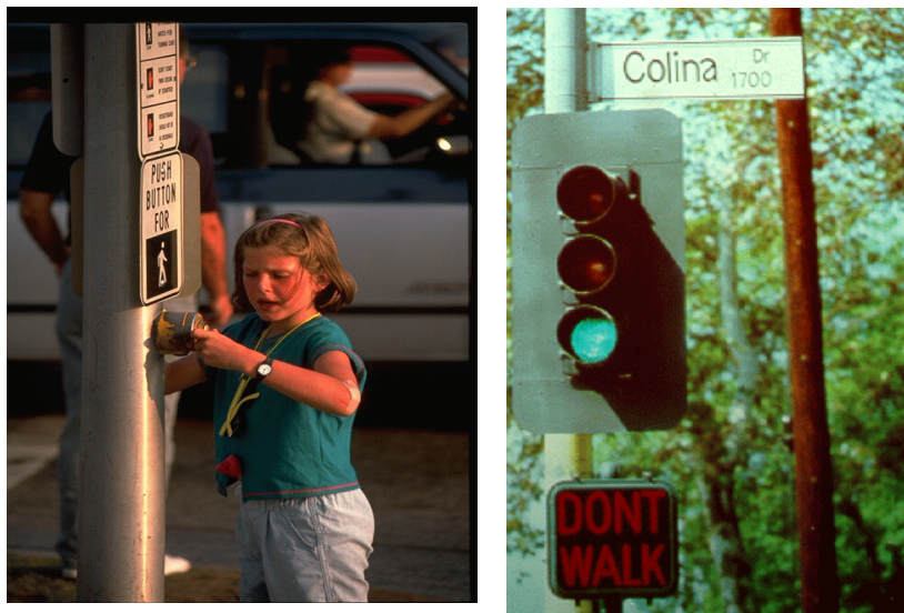
Figure 11. On some high-volume or multi-lane roads, traffic and pedestrian signals are needed to better accommodate pedestrian crossings.
