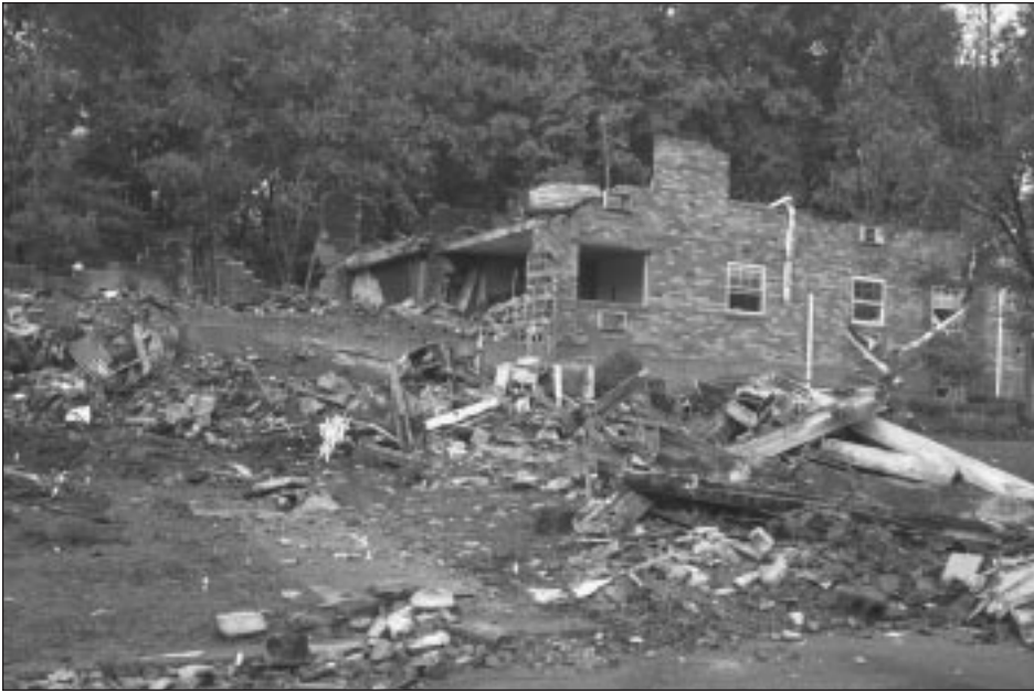
Floodwaters dislodged a gas dryer at this apartment complex, causing a gas line to explode.
