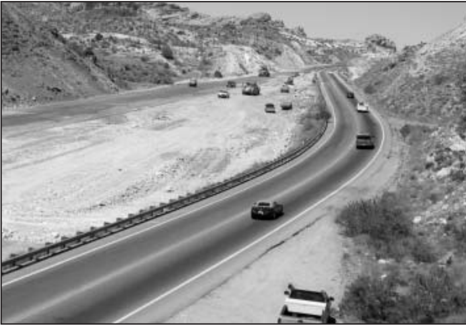
Figure 2 – Construction Along the Steep Grade on State Route 68
