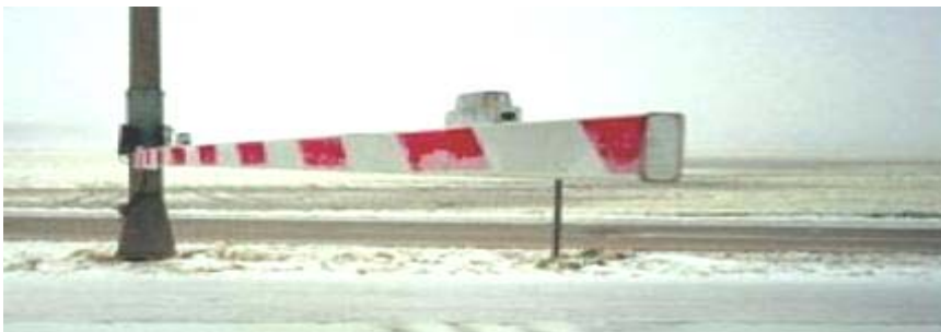
Figure 10-23: Vertical Swing Arm Traffic Gate (Closed Position) 78
