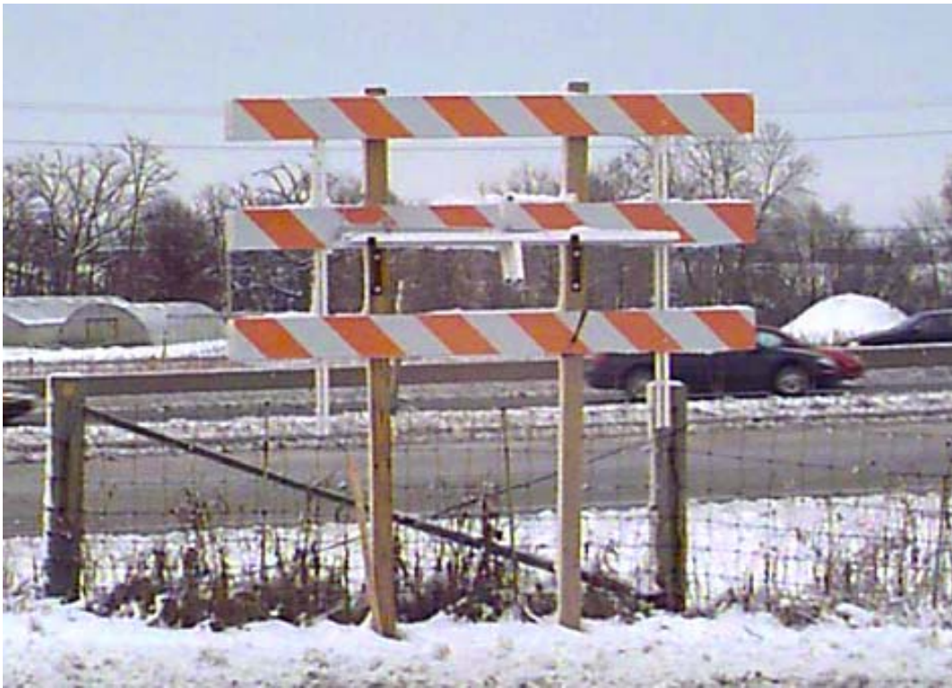
Figure 10-20: Type III Barricade (Stored Position) 77
