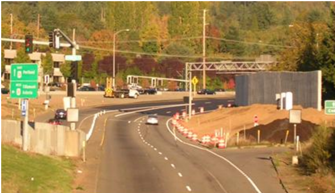
Figure 10-4: Example of Freeway-to-Freeway Metering
