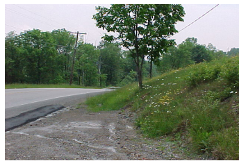
Before slope flattening
