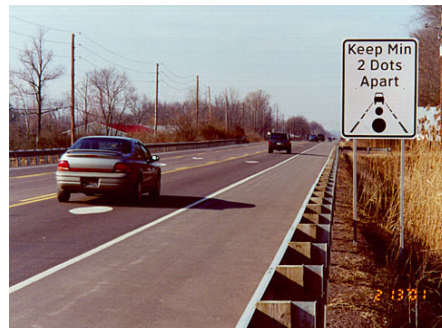
Dot treatment signage indicates safe following distances.
