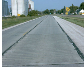
Rumble warning panel
