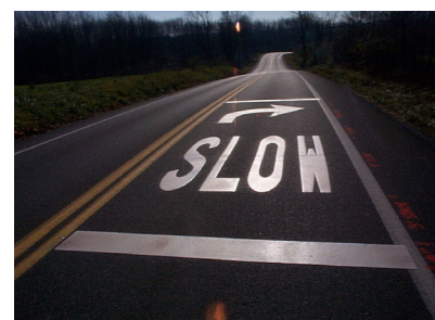
The advanced curve warning treatment warns drivers to reduce speeds.
