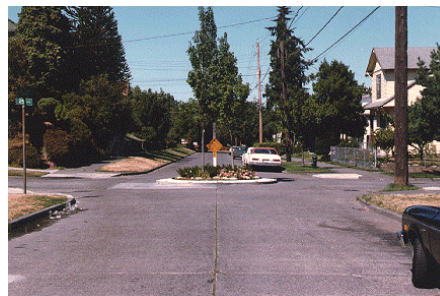
Portland has used traffic circles like the one shown above for approximately five years, dramatically reducing multi-vehicle crashes.
