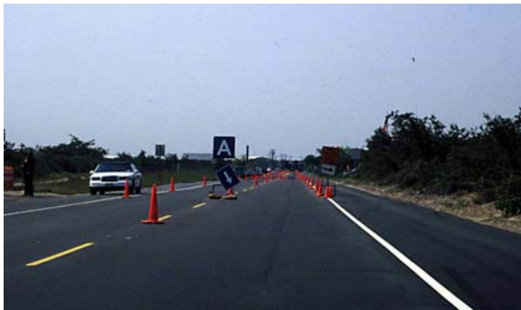
Figure 6-9 Shoulder Utilization
