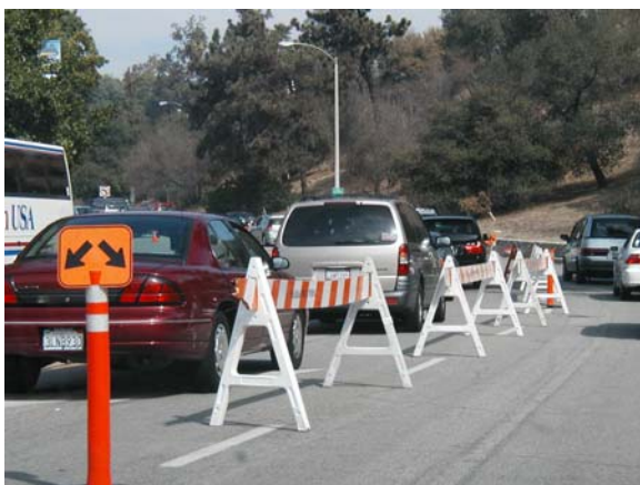
Figure 6-10 Lane Channelization
