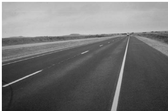
FIGURE 19-7 Asphalt bleeding in travel lane.
