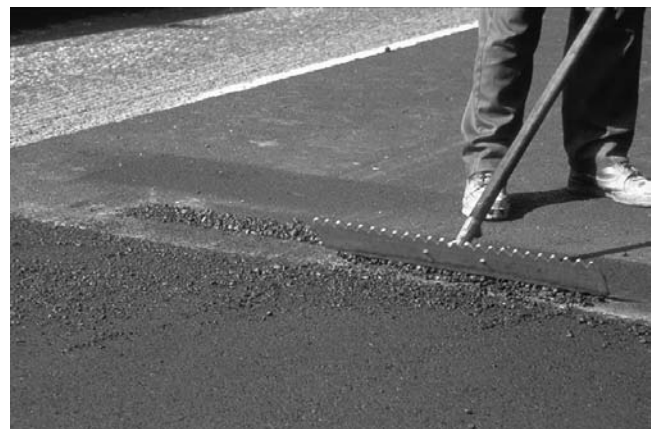
FIGURE 17-6 Raking of transverse joint.
