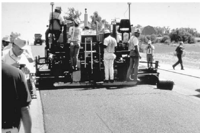
FIGURE 17-17 Compaction of mix in wedge joint.
