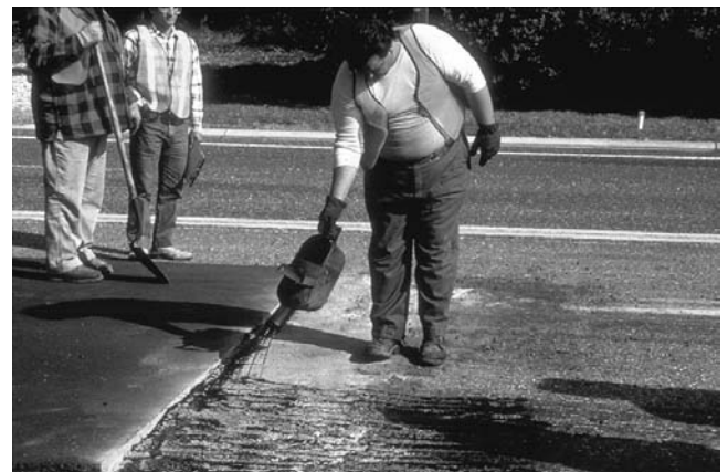
FIGURE 17-3 Application of tack at butt joint.
