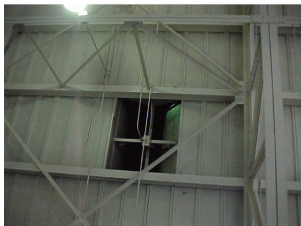
Exhibit #14. Open Roof Vents
