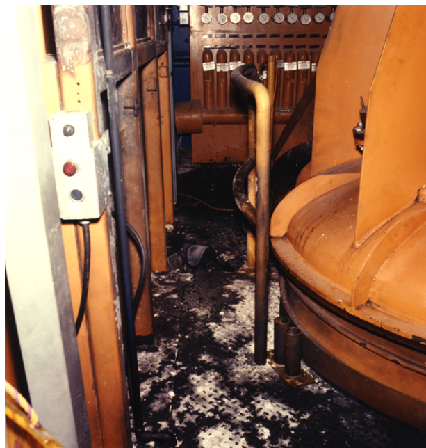
Exhibit #7. Residual NaK from Explosion Near Furnace
