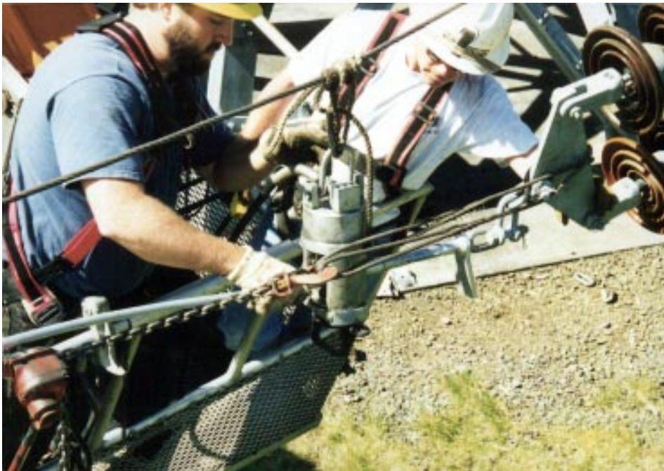
Photo 9&10 The hydraulic press is being used to permanently attach the fitting to the conductor. The hydraulic press is being operated with a press motor located in the aerial lift. The press motor operates the hydraulic system at approximately 10,000 p.s.i.
