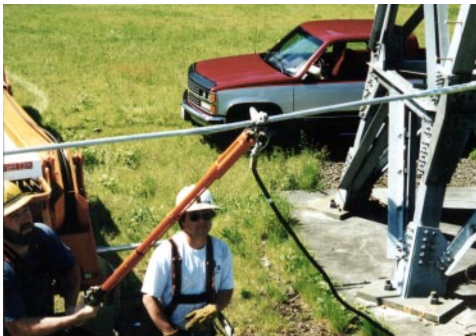
Photo F The worker is securing the clamp to the conductor. Work may now safely proceed on the conductor.
