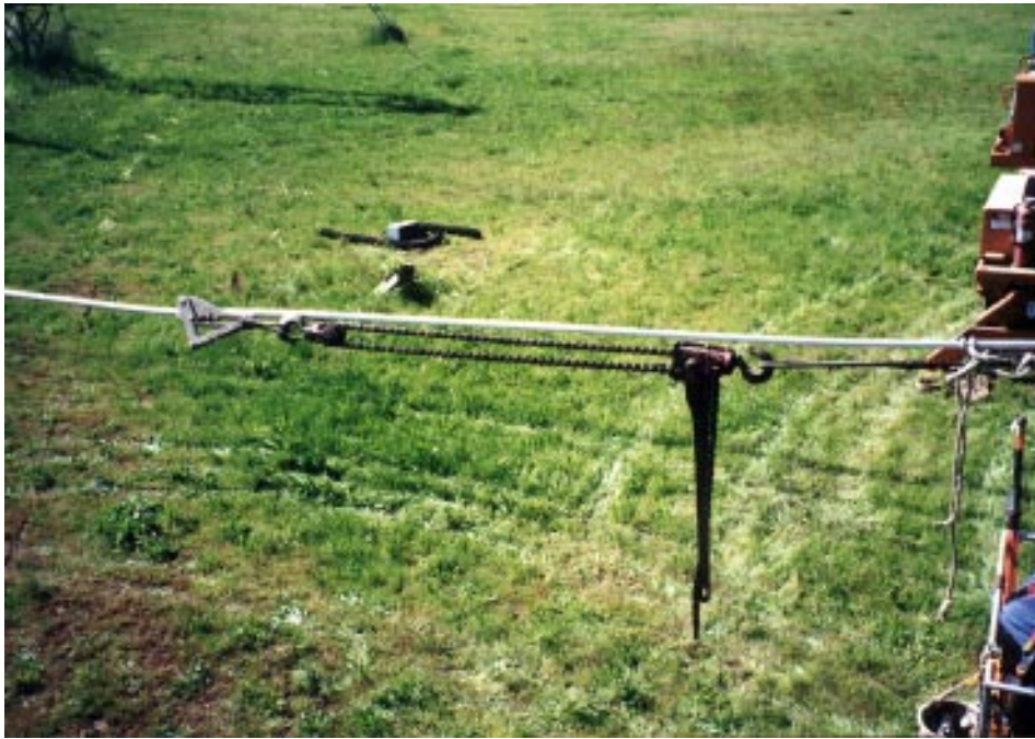
Photo 1&2 This main rigging assembly consists of a conductor grip, a hoist or come-along, and a wire rope sling terminated at the structure. This assembly is used to temporarily hold the conductor in place until the aerial crew makes a permanent connection to the tower.
