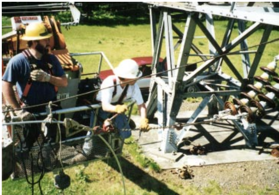
Photo 3&4 The aerial crew is in an aerial lift or “bucket”. In this initial procedure the workers are preparing to bring together the conductor and the string of insulators. This process is necessary to ensure that an accurate measurement of the conductor can be made.
