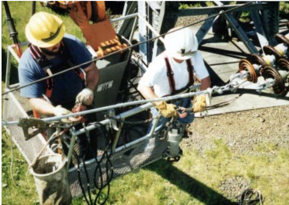
Photo 14 The crew now moves back to the main assembly (ref. photos 1&2) that was used to temporarily attach the conductor to the tower. The crew member is releasing the tension on the hoist, allowing the just completed dead end assembly to take the full tension of the line.
