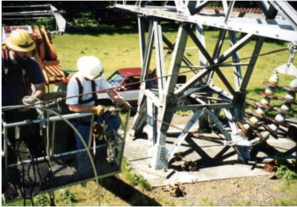
Photo 3&4 The aerial crew is in an aerial lift or “bucket”. In this initial procedure the workers are preparing to bring together the conductor and the string of insulators. This process is necessary to ensure that an accurate measurement of the conductor can be made.
