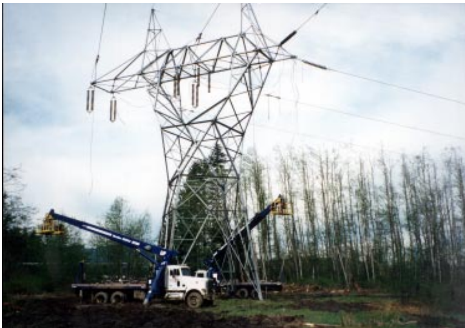
Exhibit 2 — Side View of Cranes Positioned Beneath Tower
