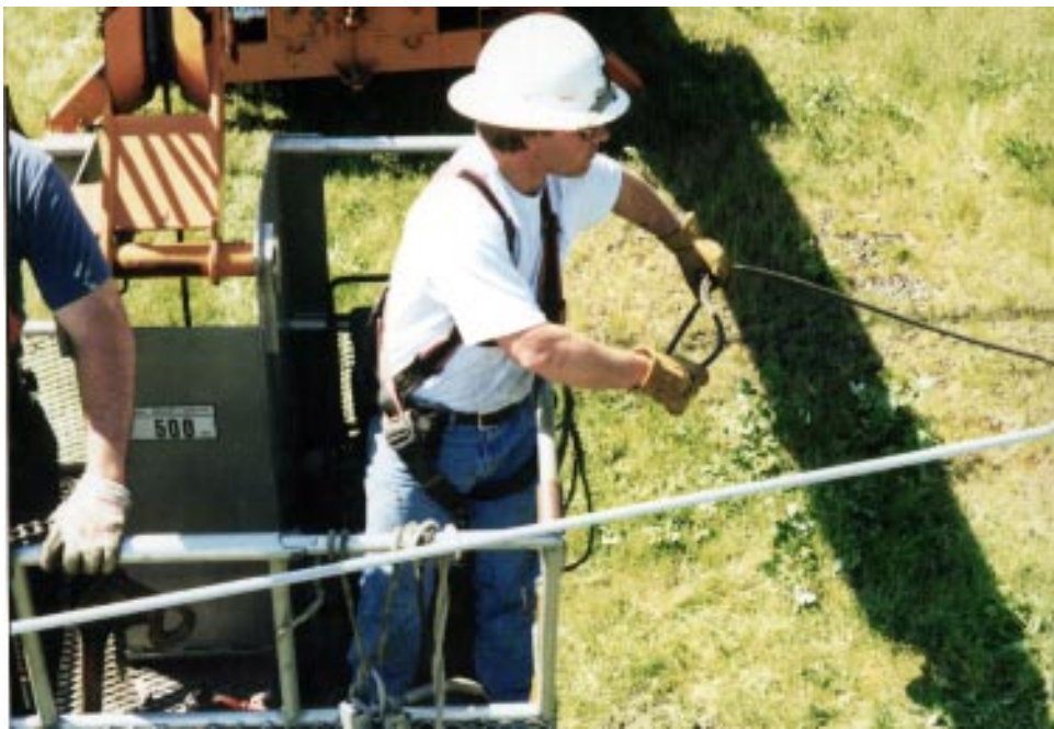
Photo 16 The worker is preparing to drop out the wire rope sling into the tower. The sling will be removed from the tower before the crew returns to the ground.
