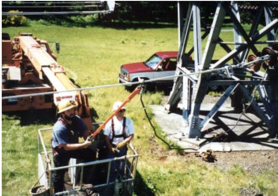
Photo F The worker is securing the clamp to the conductor. Work may now safely proceed on the conductor.
