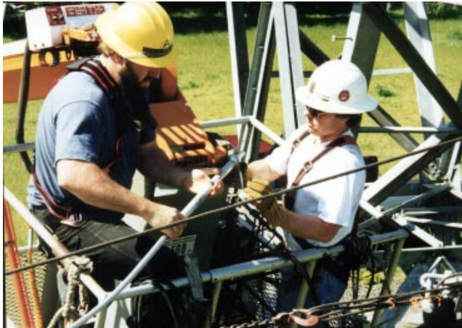
Photo 8 The worker is cutting away the outer aluminum strands of the conductor to expose the steel core in preparation of pressing on the terminal assembly. The steel core will be pressed into a steel sleeve. This sleeve is part of the complete terminal fitting.
