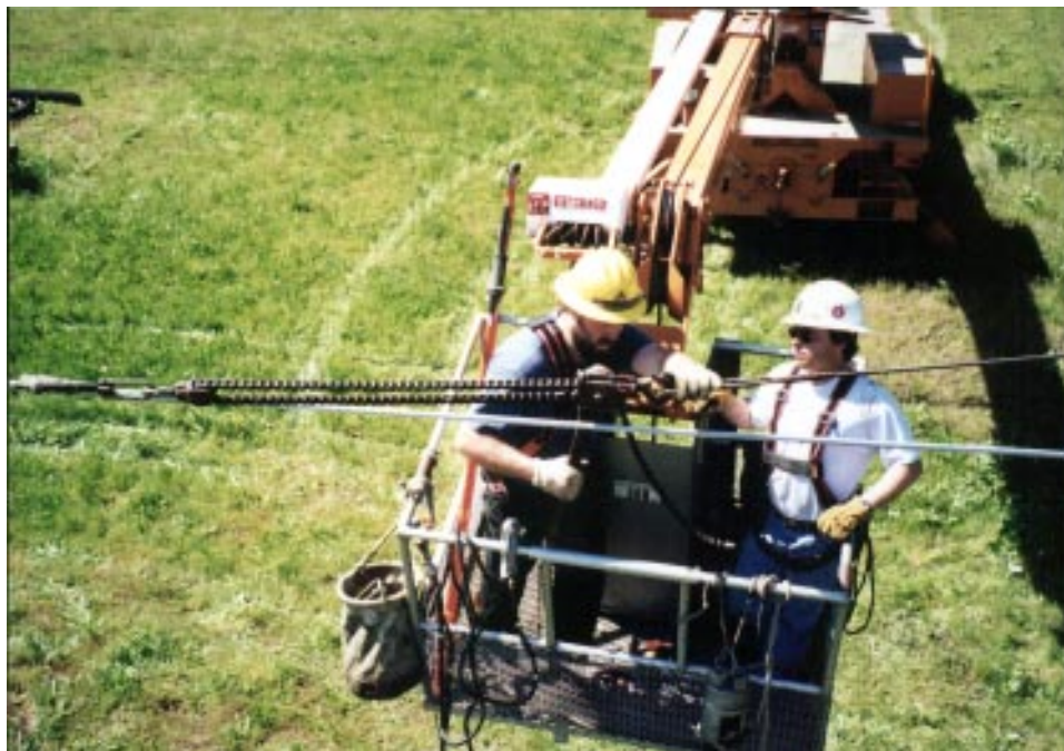
Photo 14 The crew now moves back to the main assembly (ref. photos 1&2) that was used to temporarily attach the conductor to the tower. The crew member is releasing the tension on the hoist, allowing the just completed dead end assembly to take the full tension of the line.
