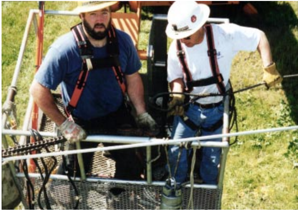
Photo 16 The worker is preparing to drop out the wire rope sling into the tower. The sling will be removed from the tower before the crew returns to the ground.
