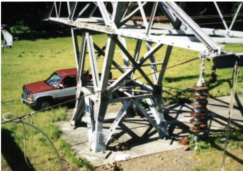
Photo 1&2 This main rigging assembly consists of a conductor grip, a hoist or come-along, and a wire rope sling terminated at the structure. This assembly is used to temporarily hold the conductor in place until the aerial crew makes a permanent connection to the tower.
