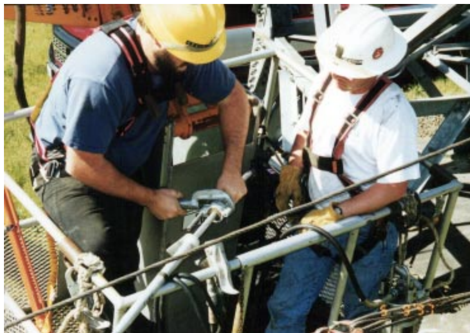
Photo 8 The worker is cutting away the outer aluminum strands of the conductor to expose the steel core in preparation of pressing on the terminal assembly. The steel core will be pressed into a steel sleeve. This sleeve is part of the complete terminal fitting.
