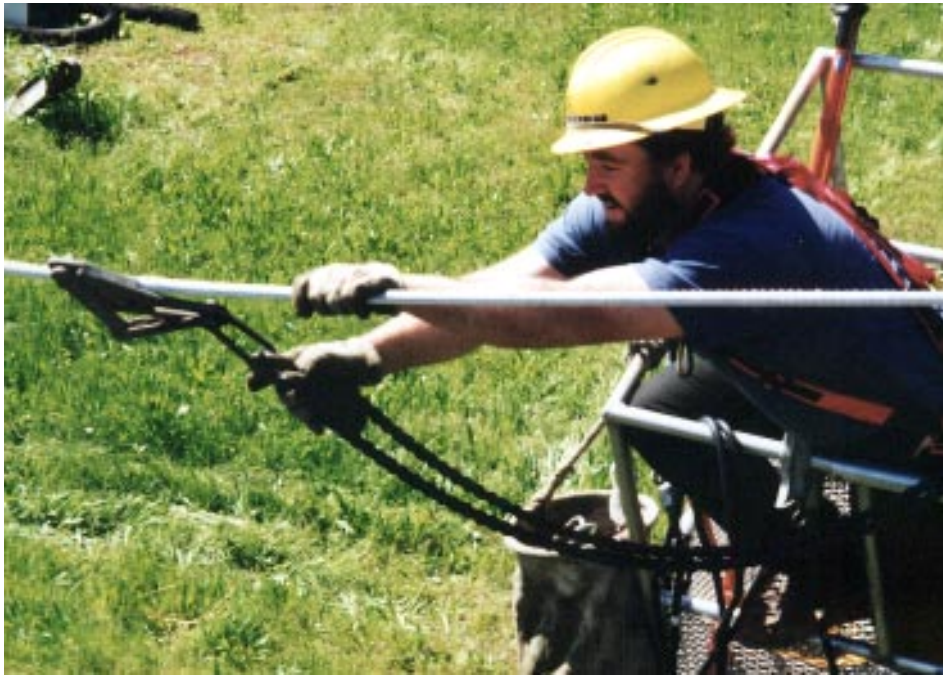
Photo 20 The hoist is removed and the last step will be to remove the conductor grip.
