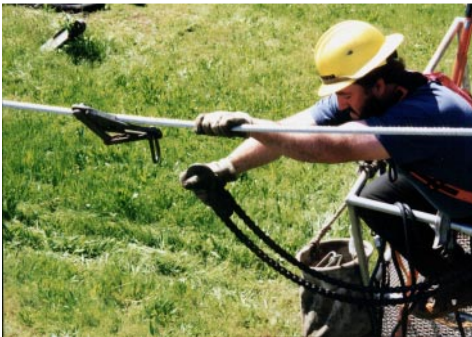
Photo 20 The hoist is removed and the last step will be to remove the conductor grip.
