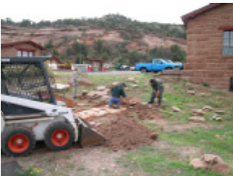
Trail rehabilitation at Colorado National Monument
