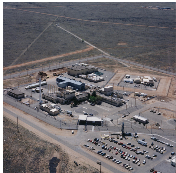
Aerial View of Technical Area V
