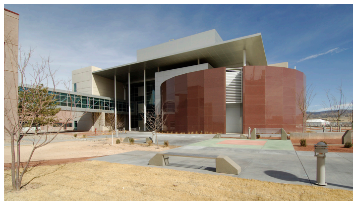
MicroFab Facility at SNL
