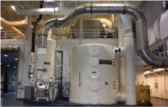
Decontamination and Waste Treatment Facility at LLNL
