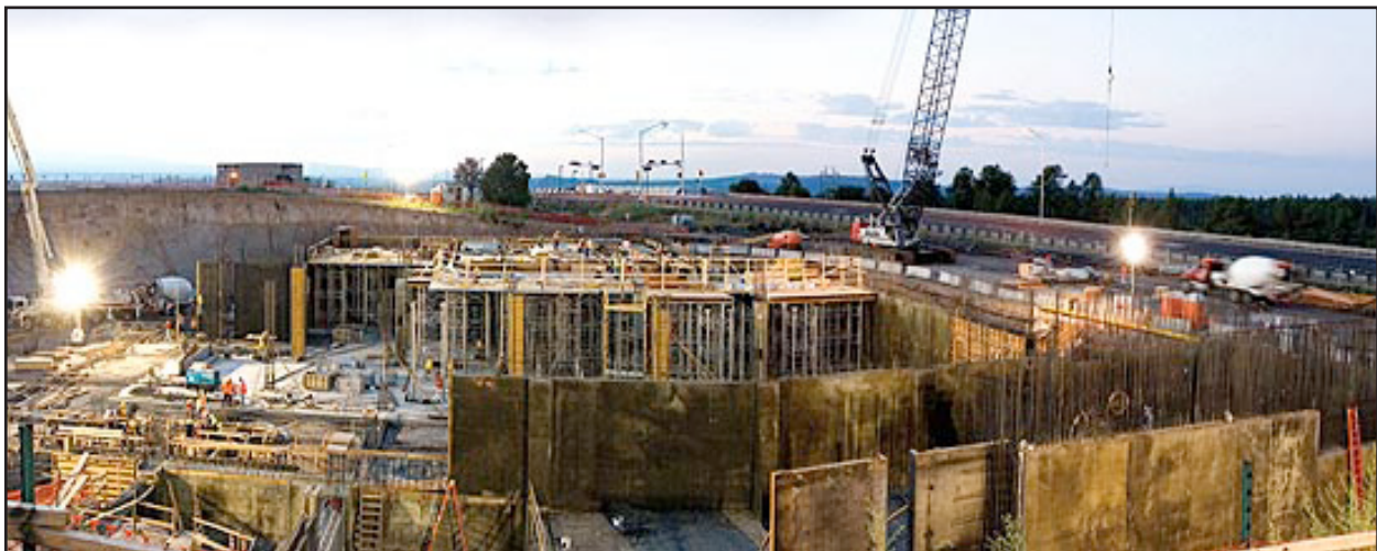
Construction site at LANL
