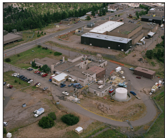
Aerial view of Radioactive Liquid Waste Treatment Facility
