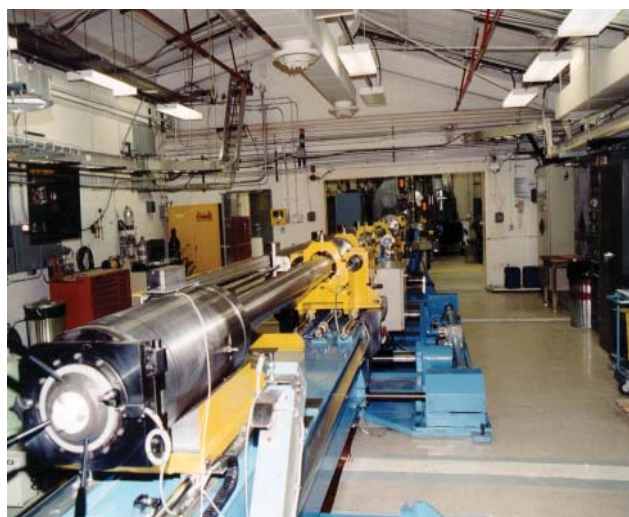
Equipment at JASPER
