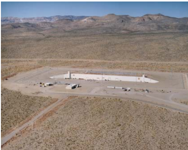
Aerial View of DAF
